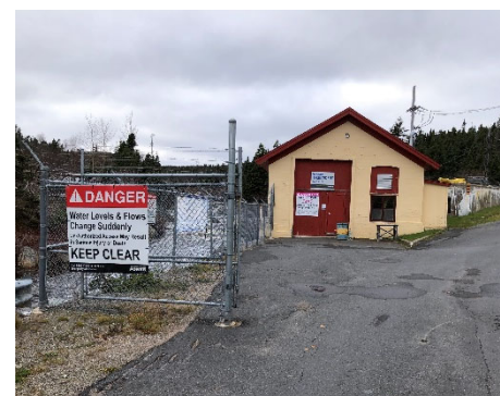
Port Union Hydroelectric Generating Plant.
