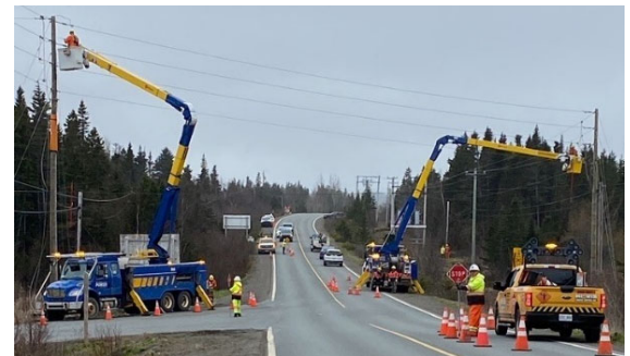
Construction on SUM-01 distribution feeder project.
