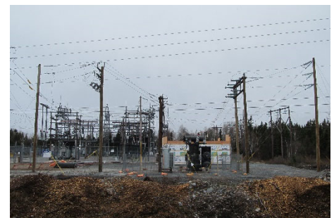
Construction at Gambo Substation in Central Newfoundland.
