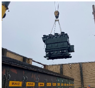
Transformer removal at Memorial Substation in St. John's.
