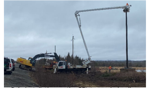
Pole installation on the 55L transmission line rebuild project.
