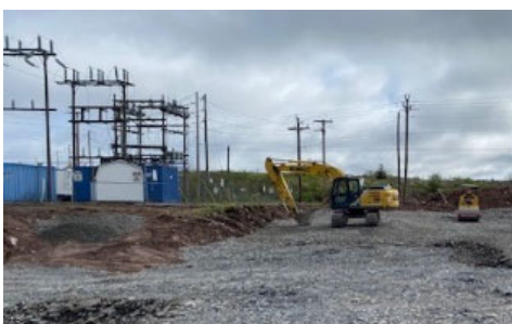
Construction at Old Perlican Substation on the Avalon Peninsula.
