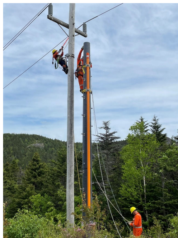
Crews in St. John's Region installing a composite transmission line pole.
